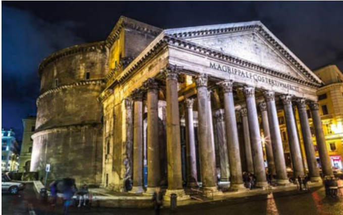
Fig. 1.5 Roman Pantheon —The first concrete building believed to be built in the world. The building has a largest unreinforced solid concrete dome (43.3 m diameter) built at that times. The building has sections large enough to keep the stress level in its different components sufficiently small to withstand the loads ( Source Internet)
