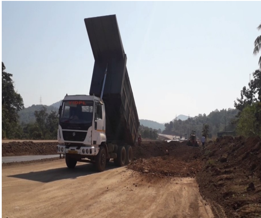
Figure 4.4: Truck dumping soil at ch.90+200
