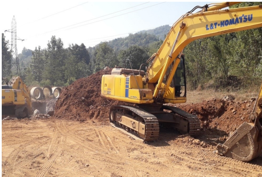
Figure 4.1: Excavator working at ch. 90+53
