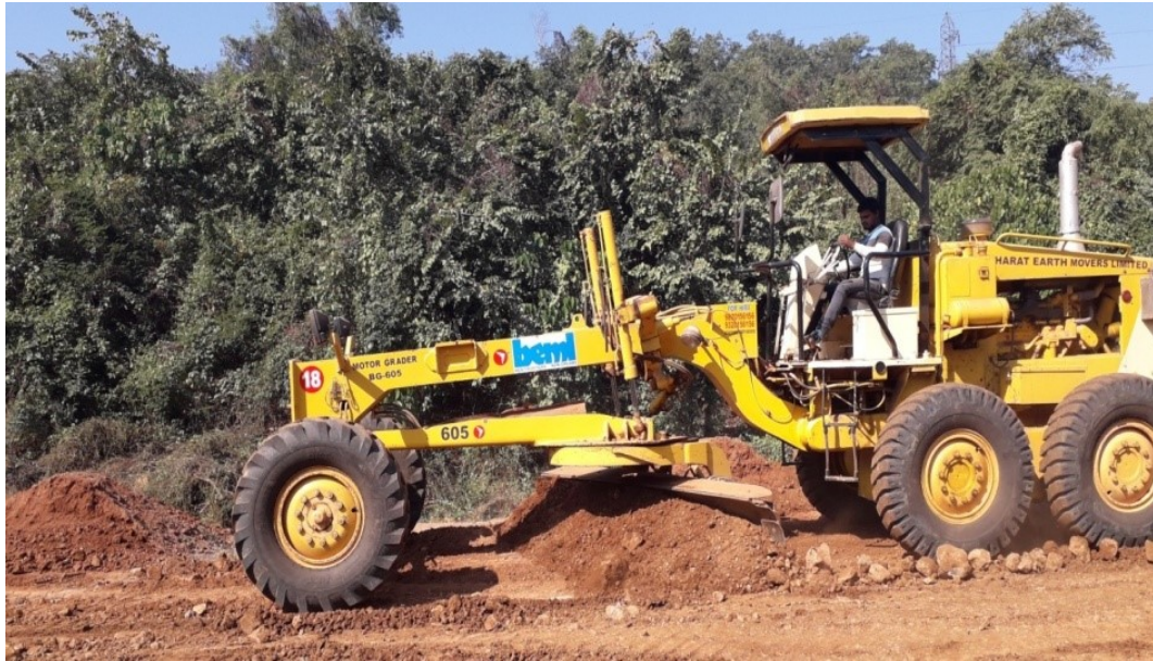
Figure 4.2: Grader spreading soil at ch.90+100
