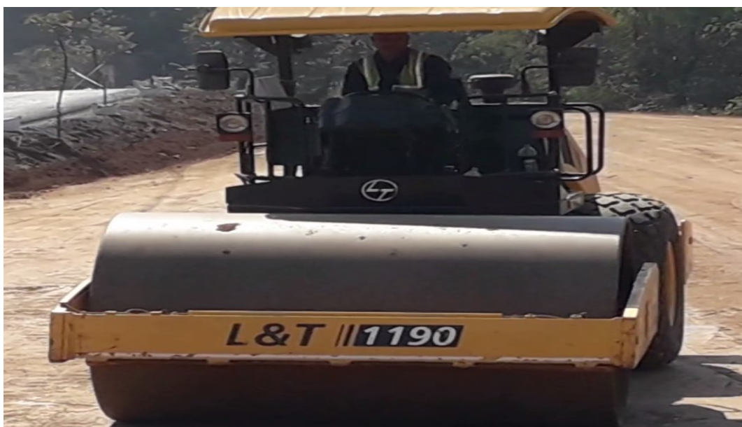
Figure 4.3: compactor spreading soil at ch.90+880
