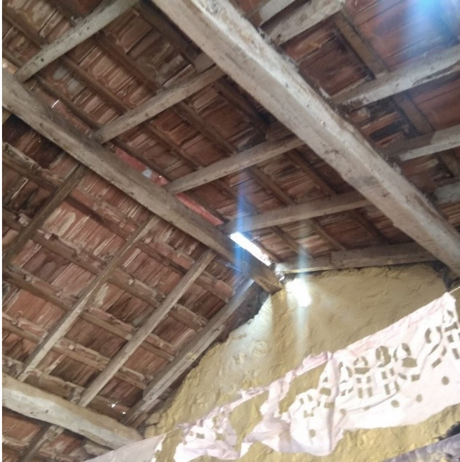
Figure 5.2: Breaking of manglorian tiles
