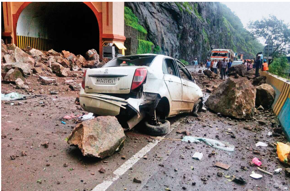
Figure 5.2: Landslide in hilly section
