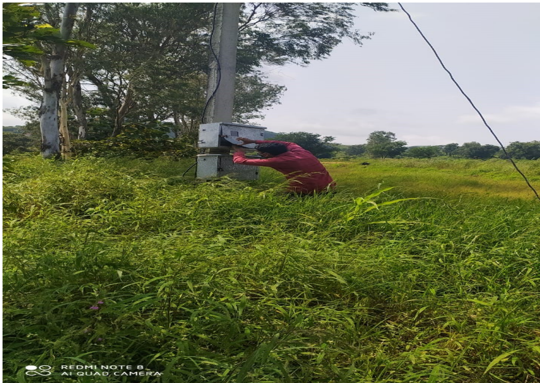
Figure 7.10: Ready for pumping test
