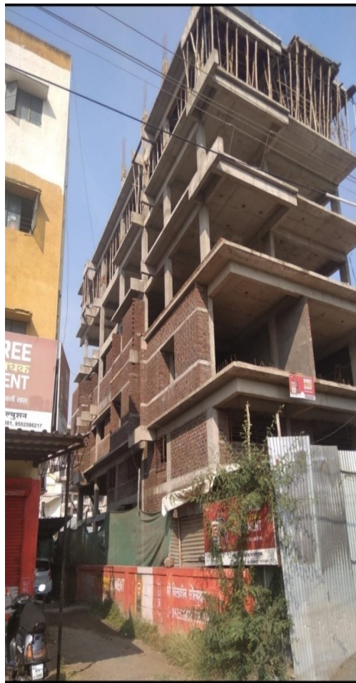
Figure 5.1: Site picture ongoing construction
