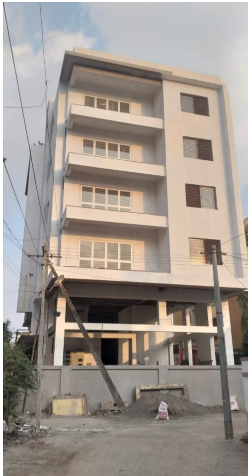
Figure 5.2: Site Picture after the completion of building
