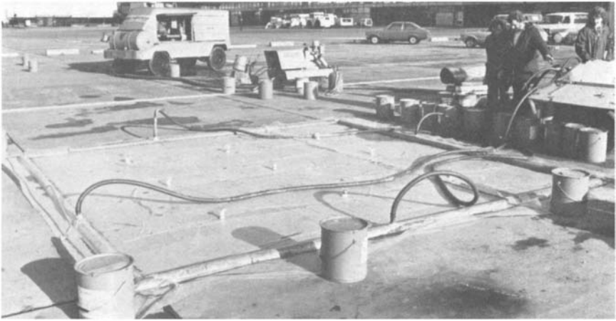
Figure 12.15 Grouting voids under concrete paving slab, and repairing cracks in slab, by Balvac vacuum injection process (BICC Ltd)
