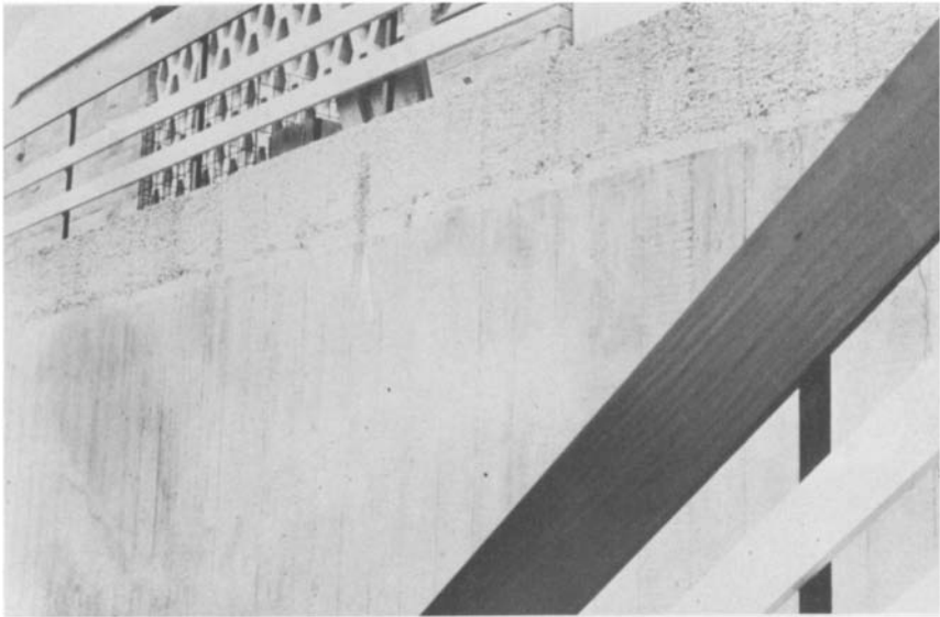
Figure 1.7 Marks of formwork joints still visible after bush hammering
