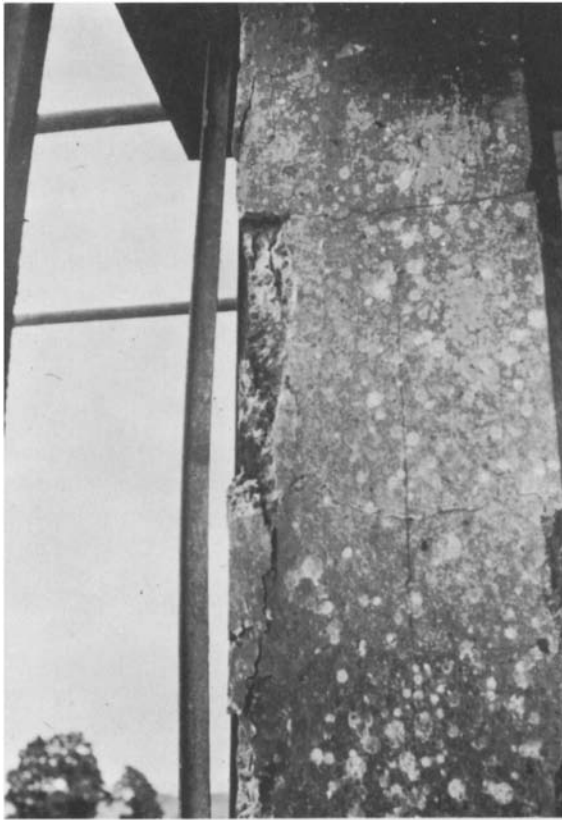
Figure 2.2(a) Reinforced concrete structure damaged by fire
