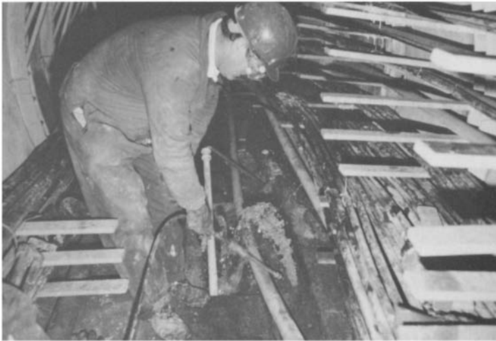
Figure 9.8 Preparing to tackle a leak from the invert of a cable tunnel
