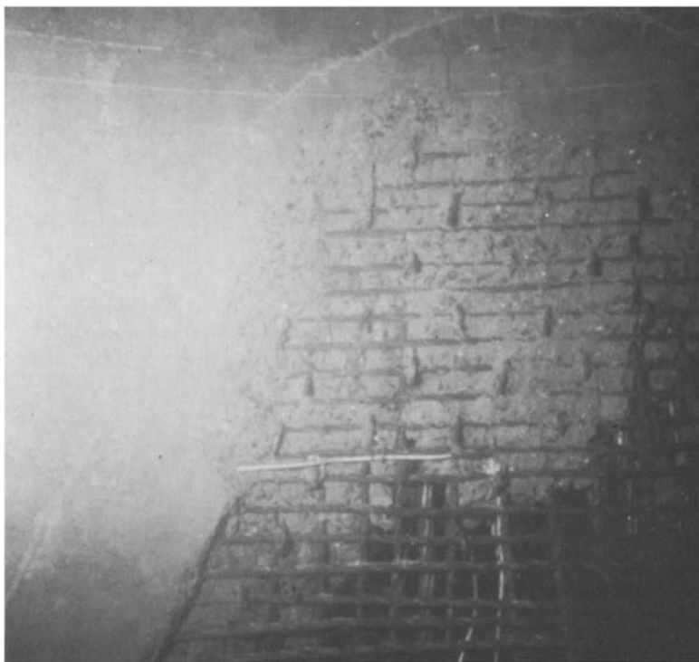
Figure 11.2 Damage caused by impact
