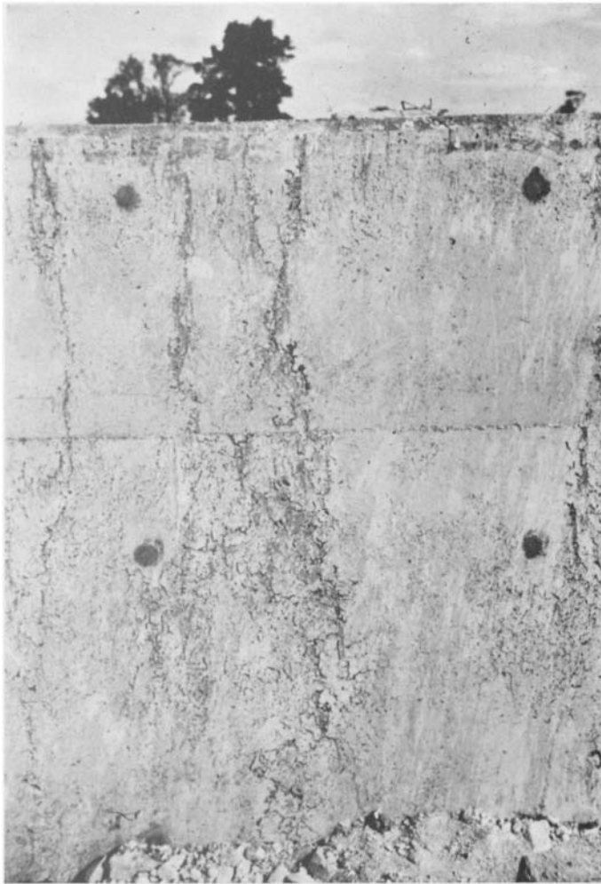
Figure 1.8 Scouring of a vertical surface caused by upward movement of water (British Cement Association)
