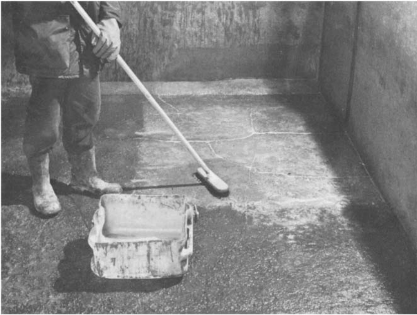
Figure 12.9 Hydrochloric acid solution being applied and pressure-washed off (British Cement Association)
