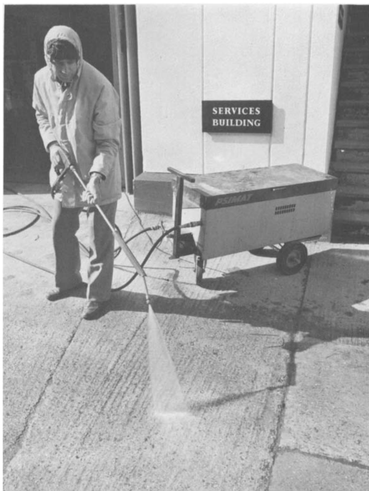
Figure 12.10 Cleaning dirty concrete with high-pressure water (British Cement Association)
