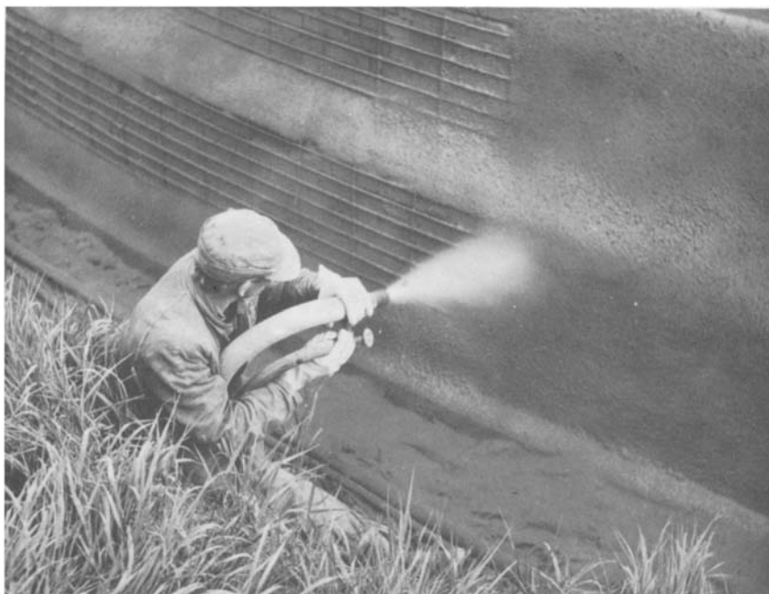
Figure 7.10 Spraying concrete to repair and strengthen settlement tank
