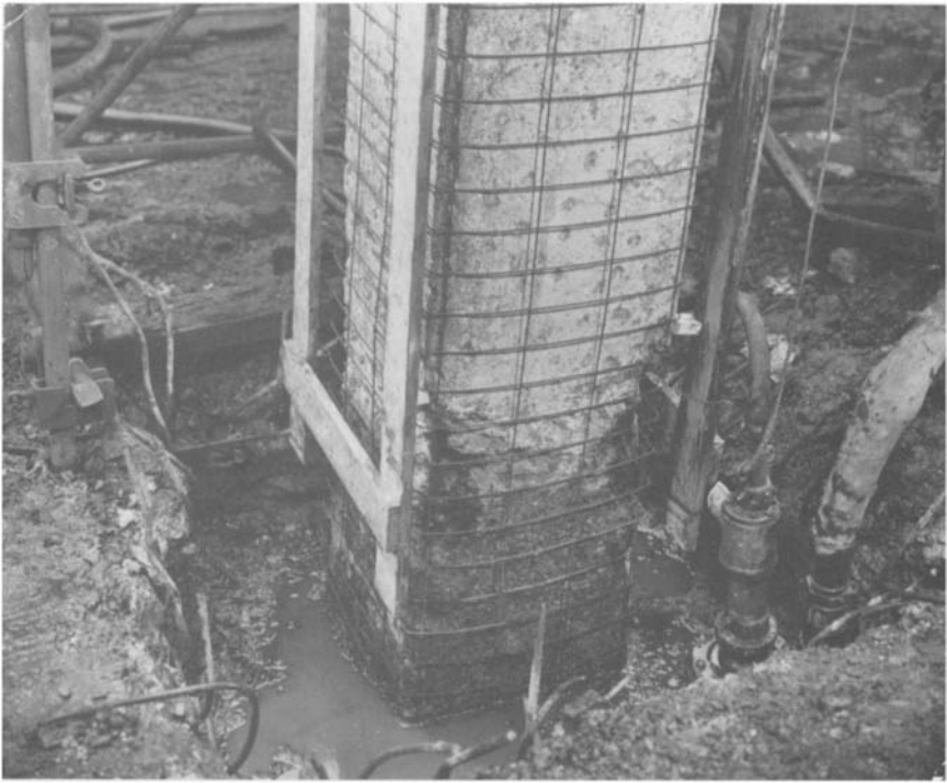
Figure 7.7 Concrete column with reinforcement and timber forms fixed for sprayed concrete repair
