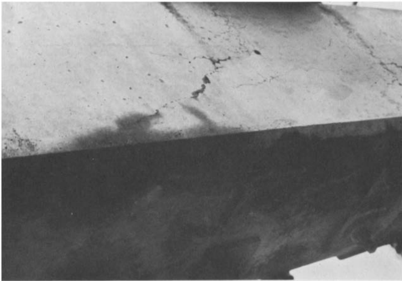
Figure 2.4 Cracking caused by freezing of water in bolt pockets
