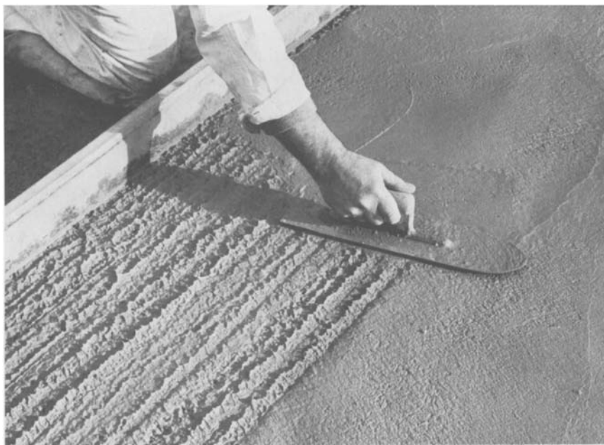
Figure 12.16 Laying of granolithic floor topping (British Cement Association)
