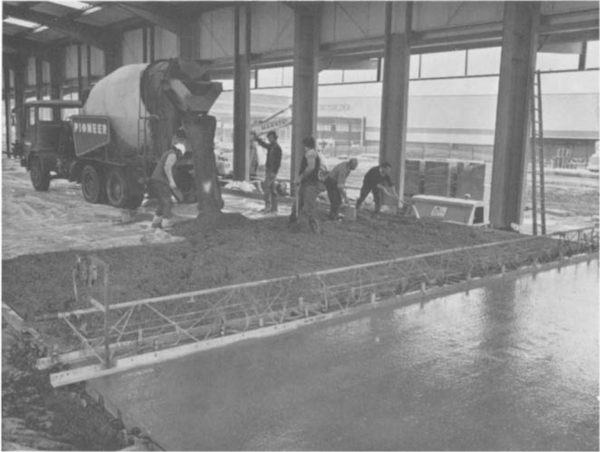
Figure 12.2 ‘Razorback’ beam being used for compacting concrete in an unreinforced concrete floor slab (British Cement Association)
