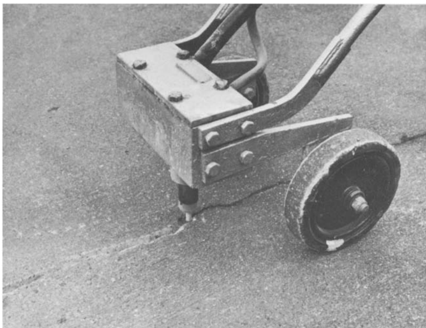
Figure 12.14 Using a crack router with 12 mm head to chase out the crack (British Cement Association)
