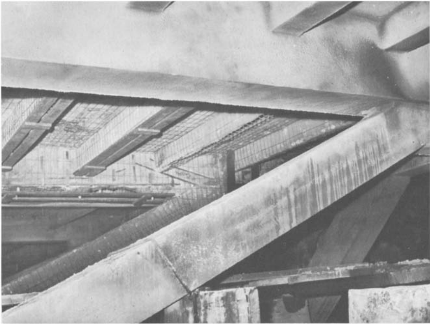
Figure 7.6 Sprayed concrete repairs to quay substructure in progress and completed
