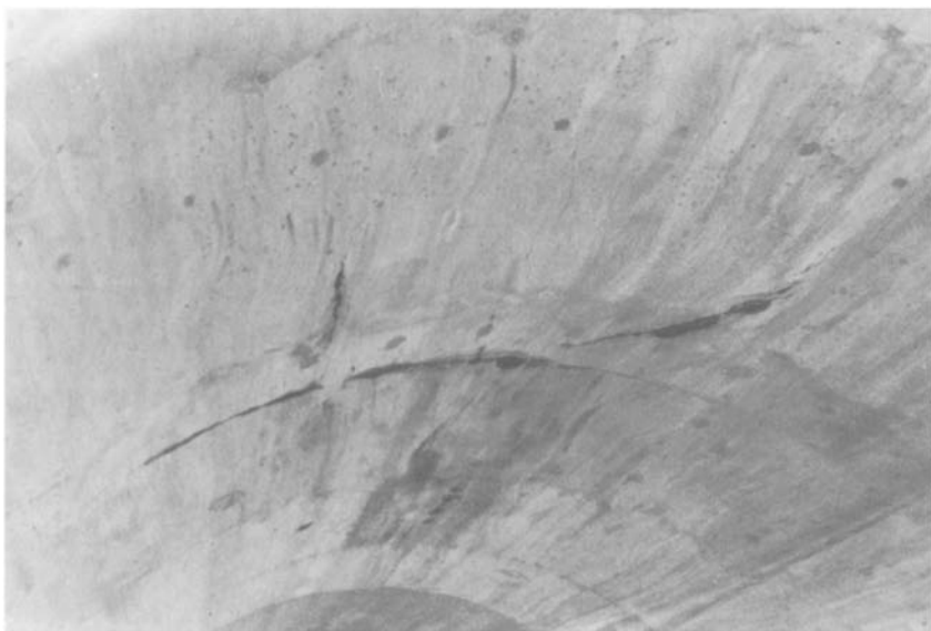
Figure 9.1 Leakage through cracks and construction joints in a concrete shaft
