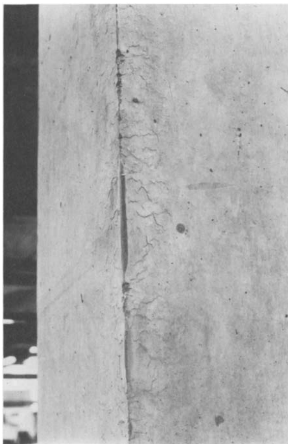
Figure 1.4 Plastic settlement cracks in arris of r.c. column inwardly sloping formwork, but their incidence is reduced if the form face is slightly absorbent. With impermeable formwork, blowholes may be a sign of inadequate vibration of the concrete but, even with good compaction, it may be difficult to avoid them altogether. Both the type of release agent used and the concrete mix design have considerable influence on the formation of blowholes—a very cohesive mix tends to produce more than a less cohesive one.
