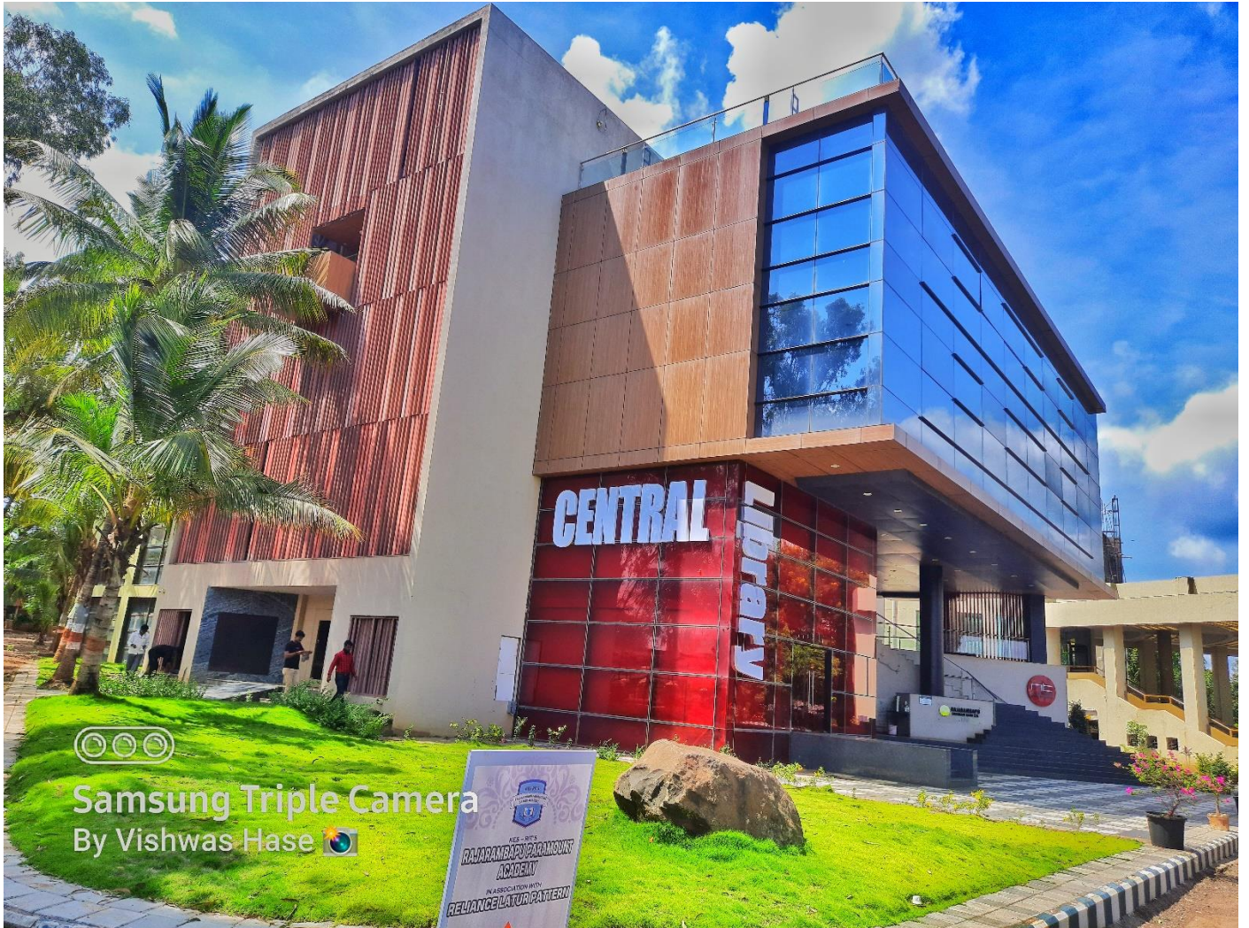
RIT CENTRAL LIBRARY BUILDING
